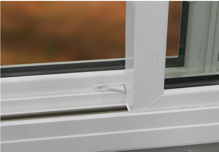
Push button spring-loaded vent latches allow both window sashes to remain partially open for ventilation.
