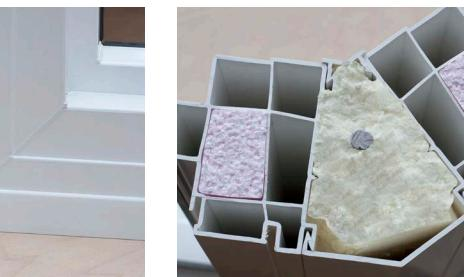
Silicone Free Interior and Exterior to improve aesthetics. Exterior drip cap.
